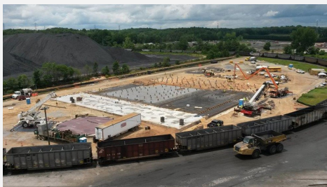
Marshall ash basin | Duke Energy
